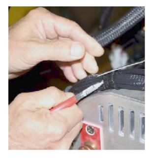
5. Cut wire 106 going to the Engine/Generator Controller after the existing connection point and install the conductors that lead to the new in-line fuse holder. Use insulated butt splice connectors for these conductors.
